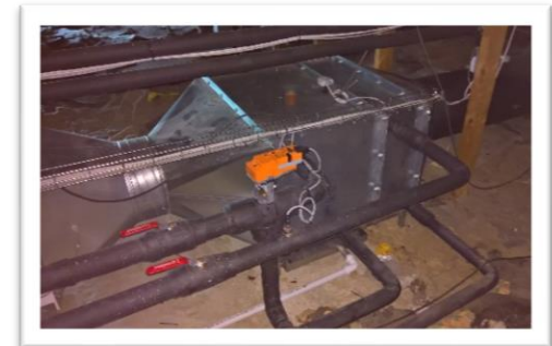
Exhaust air heat recovery pack
